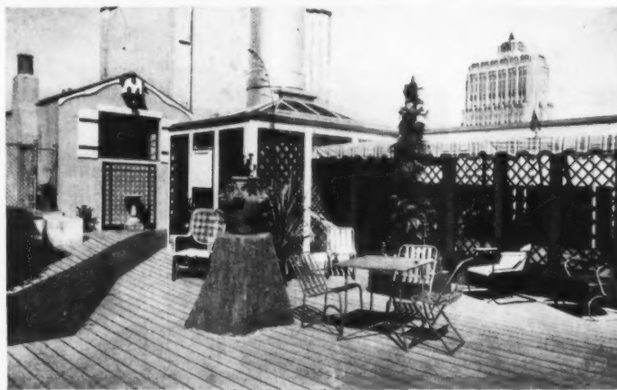
View of penthouse patio on roof of San Francisco Examiner building
